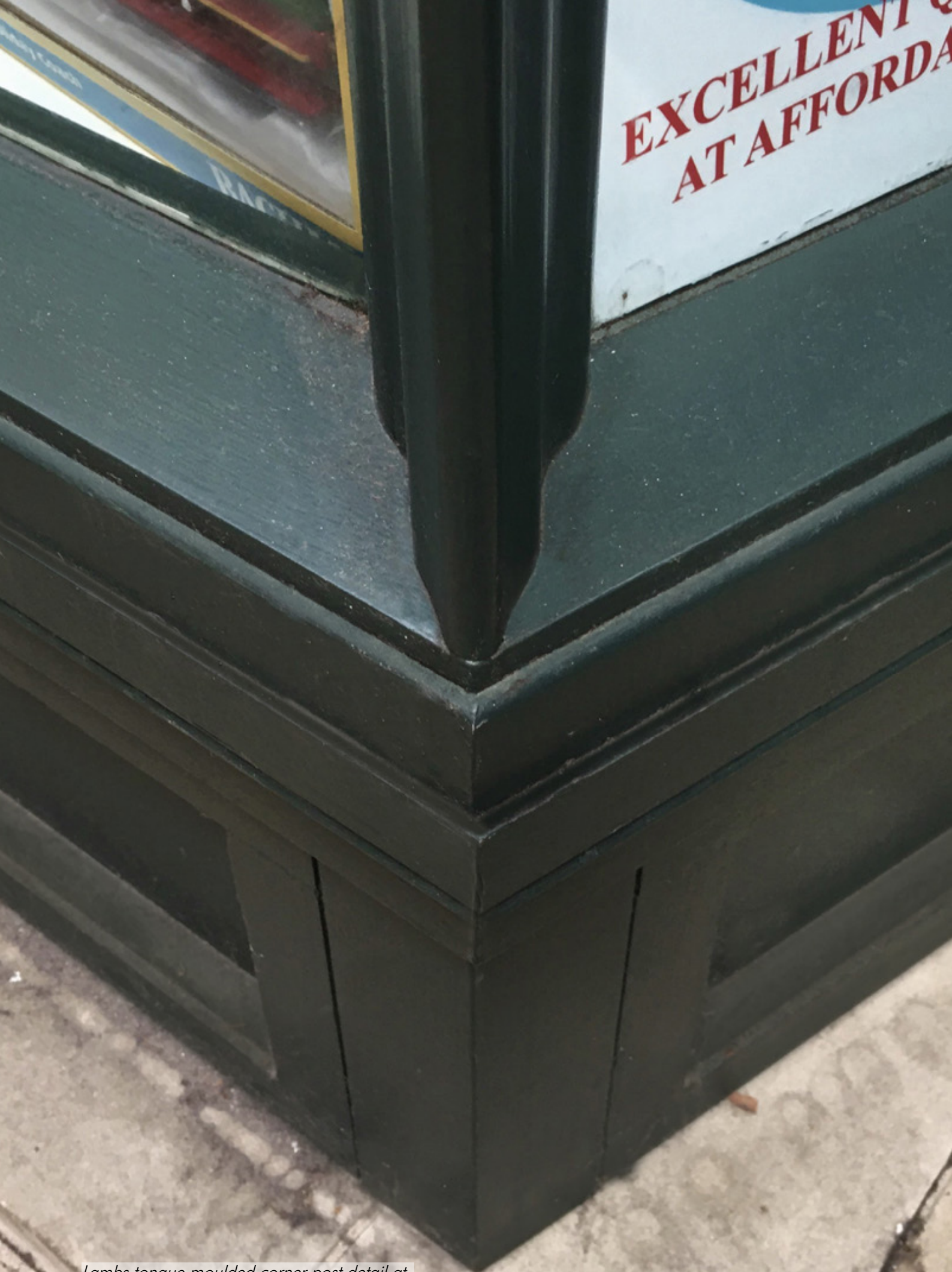
Lambs tongue moulded corner post detail at 3-4 The Strand Arcade, Derby
