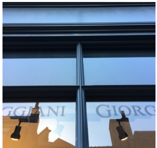
28 Sadler Gate: The project officer worked closely with the contractor to ensure a high quality 'lamb's tongue' finish to the glazing bars.
